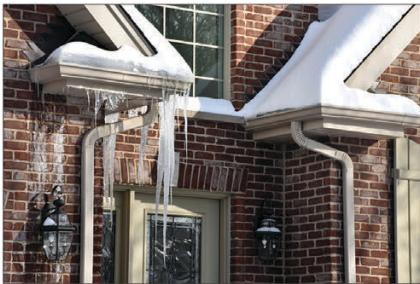
Picture above shows the Left Eave with No Gutter Drainer • Right Eave with Gutter Drainer Installed
