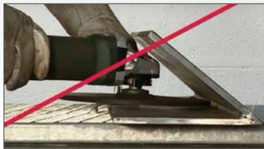
This solution violates safety standards
